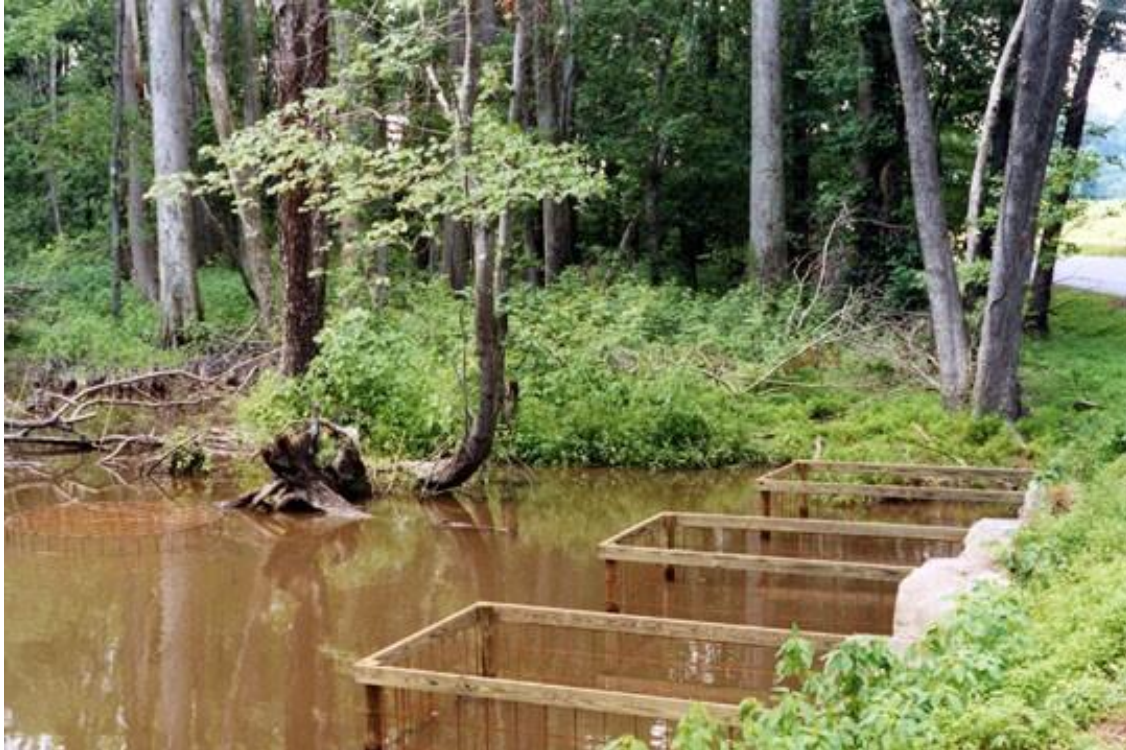
Figure 6. Three Beaver Deceivers™ installed in June 2004 to protect five culverts directing water underneath Route 644 near Lake Cohoon in the City of Suffolk, Virginia. A Round Fence™ (left center) and a Castor Master™ (beneath the surface of the water between the Round Fence™ and the center Beaver Deceiver™) were attached to the upstream end of the center Beaver Deceiver™ to augment water flow if beavers attempted to dam the fences.
